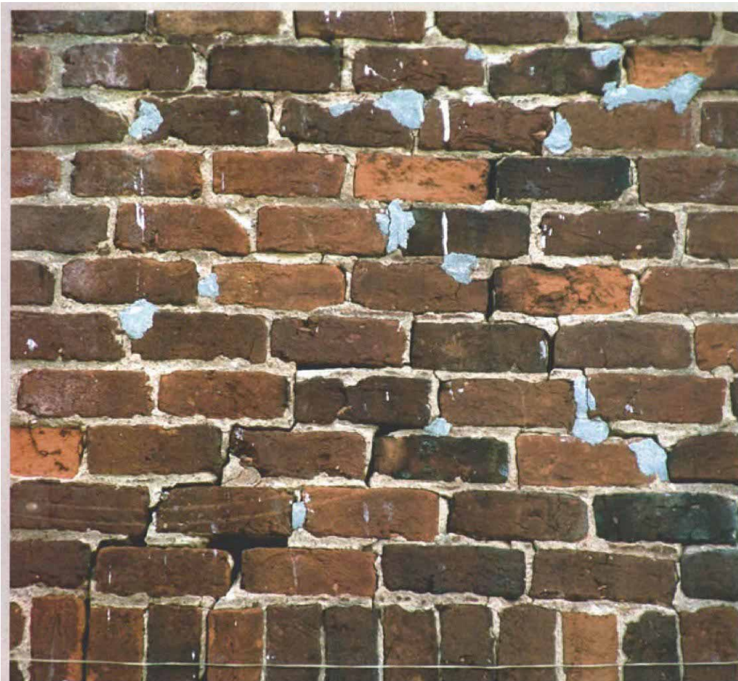
Look for continuous or zigzag cracks in masonry walls. Although small cracks are to be expected, the long, continuous cracks in this old brick wall suggest that the footing and foundation have settled.
