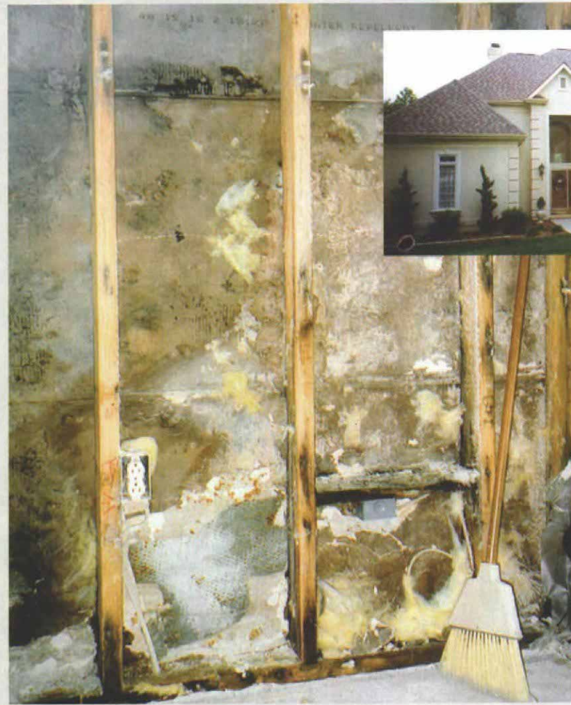
Rot lurks below. Swollen joints and cracked paint on this hardboard composite siding are signs that water has gotten in and that the material is rotting.
